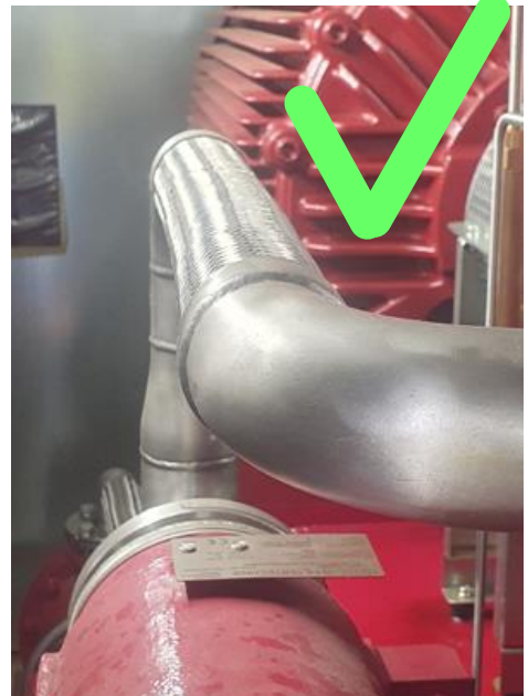
Figure 2 Same situation after repair, hose with correct length was mounted
